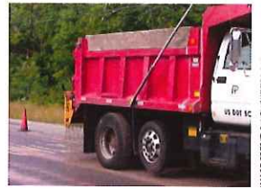
After rejuvenator placement, light coating of sand is applied to enhance friction
