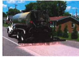
Nashville has adopted the use of pavement rejuvenators like Reclamite to protect pavement that is three to five years old: pink color typical until emulsion breaks
